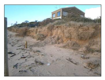
The beach between the Oliver's Hill sea wall and Frankston pier has suffered considerable erosion into the primary dune area, as shown in this photo. This winter, the total length of the beach has been severely scoured, resulting in the safety fence having to be relocated further back into the dune area, almost on to the boardwalk. The beach has been partly replenished by the dune sand, and a large proportion of this sand is now settled off the beach, forming a large sand bank at low tide level.
